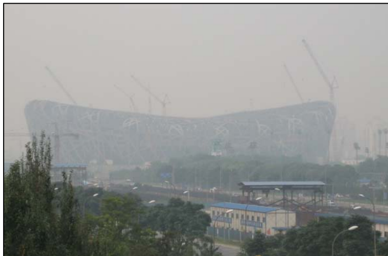
Construction of the Bird's Nest Stadium through the haze.
